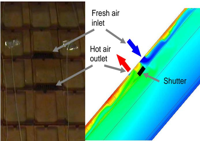
Figure 9: installation of extra openings.
