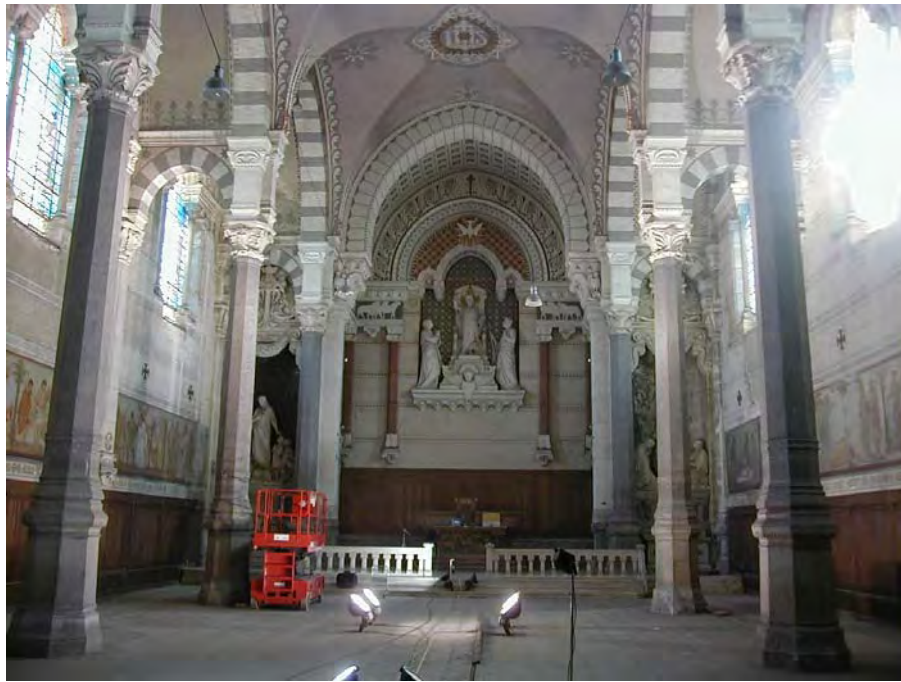
Figure 1.- Front view of the chapel
