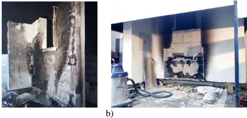
Fig. 5. View of the executed tests of ETICS with EPS. a) test with the standard plaster (7 mm about); b) test with the thick plaster layer (2 cm).
