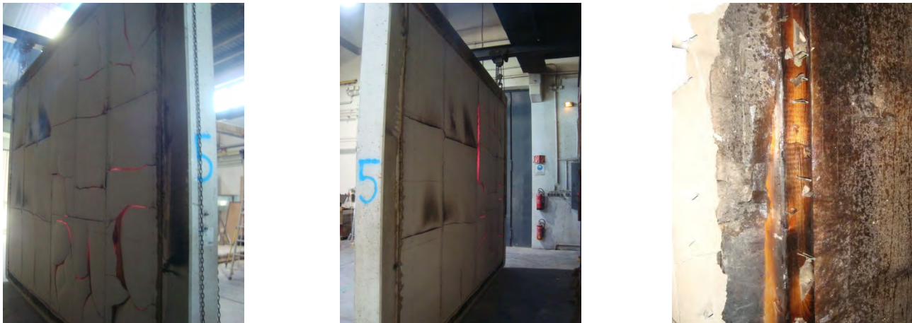
Fig. 4. a) Specimen V2: large thermal cracks b) Specimen V1: few thermal cracks in the first layer; c) Specimen V1: wooden substructure lightly charred
