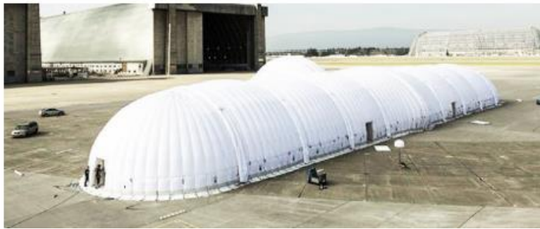
Figure 4: solar Impulse mobile hangar
