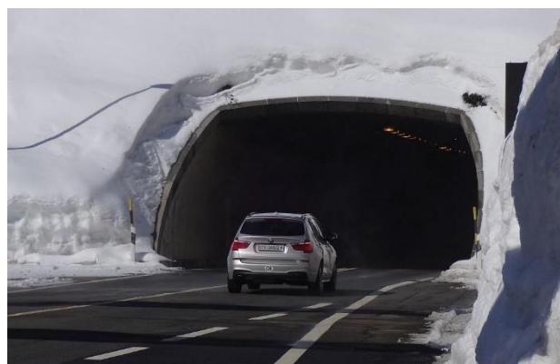
Figure 5. South entrance of the San Bernardino tunnel in winter 2014. The snow cover was removed around the sloped tunnel portal. Snow drift accumulations or new snow can easily slide (see case 3, Fig. 1). The old snow cover is stabilized by knee pines which are overfilled with snow.
