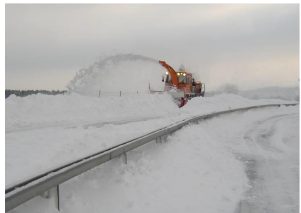
Figure 19. A75 closed to traffic: snow-removal operations
