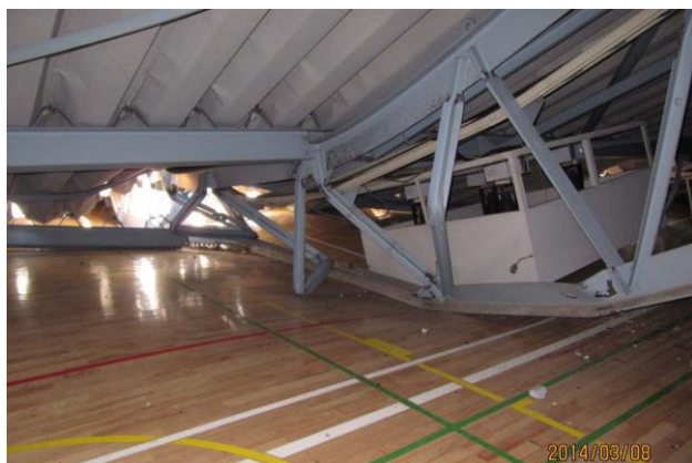
Photo 2. Internal view of Photo 1.
