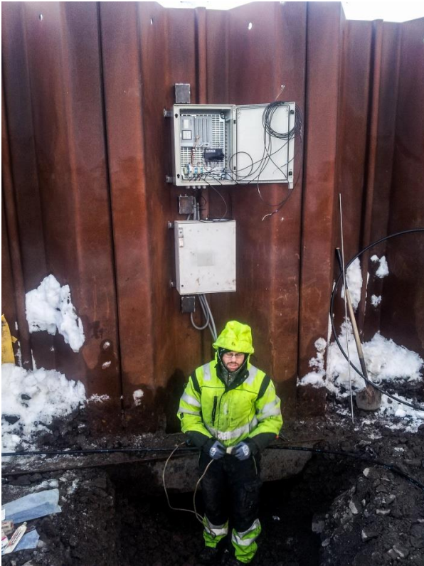
Figure 2. Installation of monitoring instruments in January 2015. Photo: MogT.
