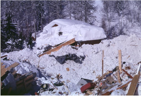
Figure 11. High pressure exerted at low velocities in the runout zone of Péclerey avalanche that hit MontRoc village (9 February 1999) – F. Rapin/IRSTEA.
