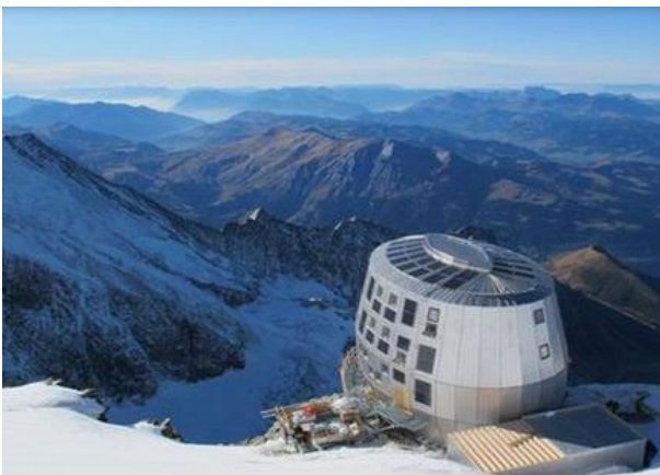
Figure 17. Melting container in the back of the building
