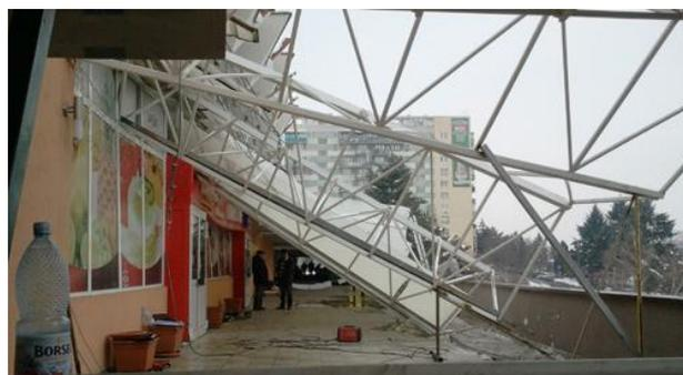
Figure 14. Collapse of a new metallic roof structure in Cluj [26]
