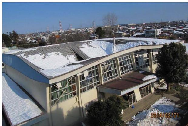
Photo 3. Example of collapsed building. (No.9 in Table 1.)
