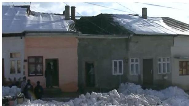
Figure 16. Collapse of an old wooden roof in Suceava [28]
