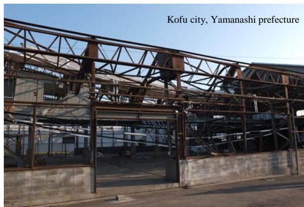
**Fig. 1** Collapse of packhouse and equipment for packing
