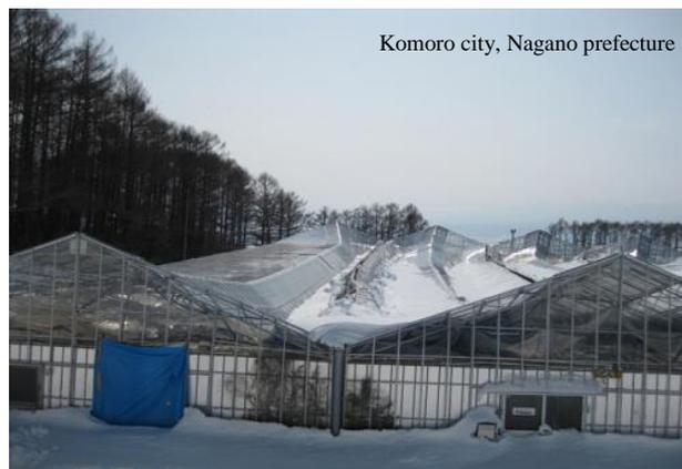
**Fig. 2** Collapse of greenhouse due to excess snow load
