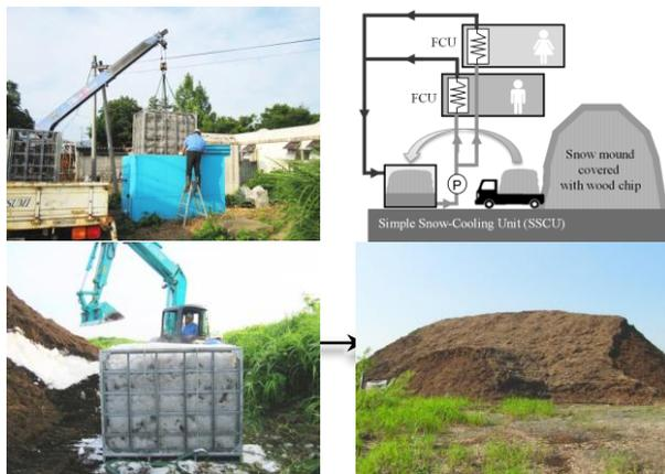
**Figure 6.** Snow cooling system for Highway SA lavatory.
