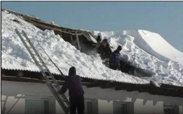
Figure 18. Collapse of a wooden roof structure in Podgoria [30]
