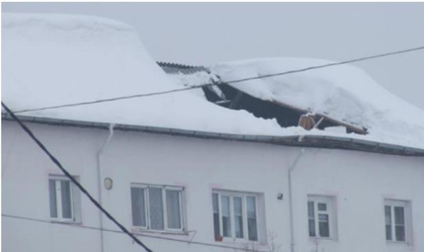
Figure 19. Collapse of a wooden roof structure in Focsani [31]
