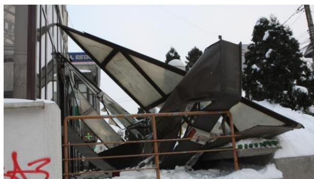
Figure 15. Collapse of a new metallic roof structure in Iasi [27]
