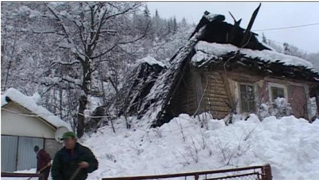
Figure 17. Collapse of a wooden roof structure in Cavnic [29]
